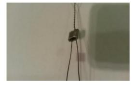
After minimum two restrictor fixing bolts fit the first ALU seal maximum 20mm after the last bolt. Then follow the instructions of the picture!
